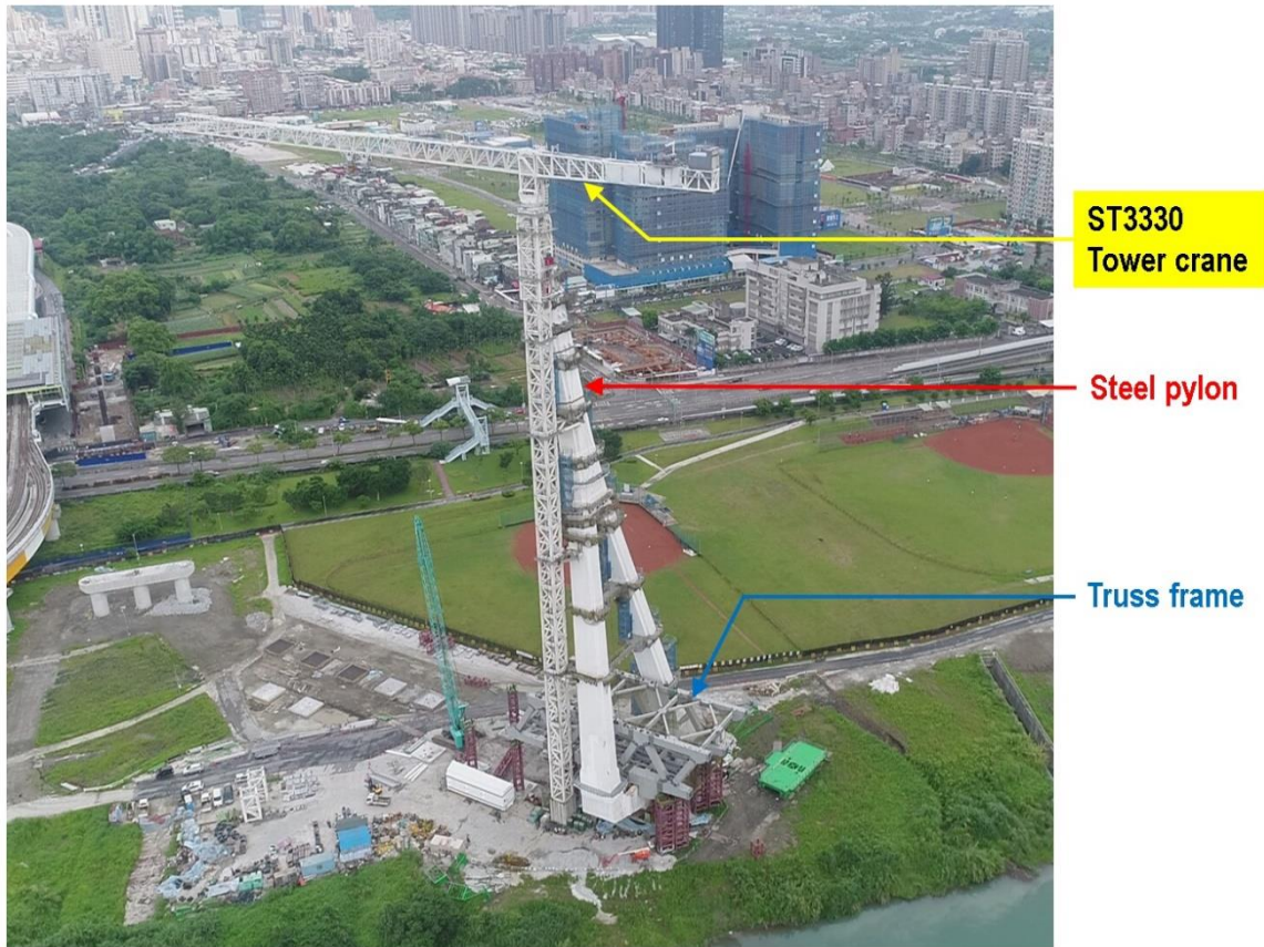
171 172 Figure 6: The photo of ST3330 tower crane
