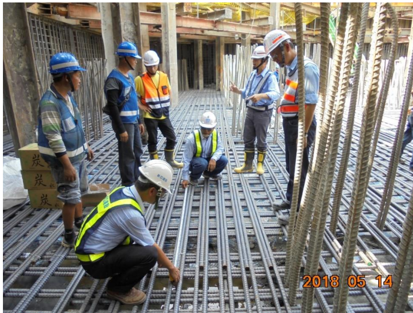
259 Figure 16: The inspection of the foundation by the QC engineers.
