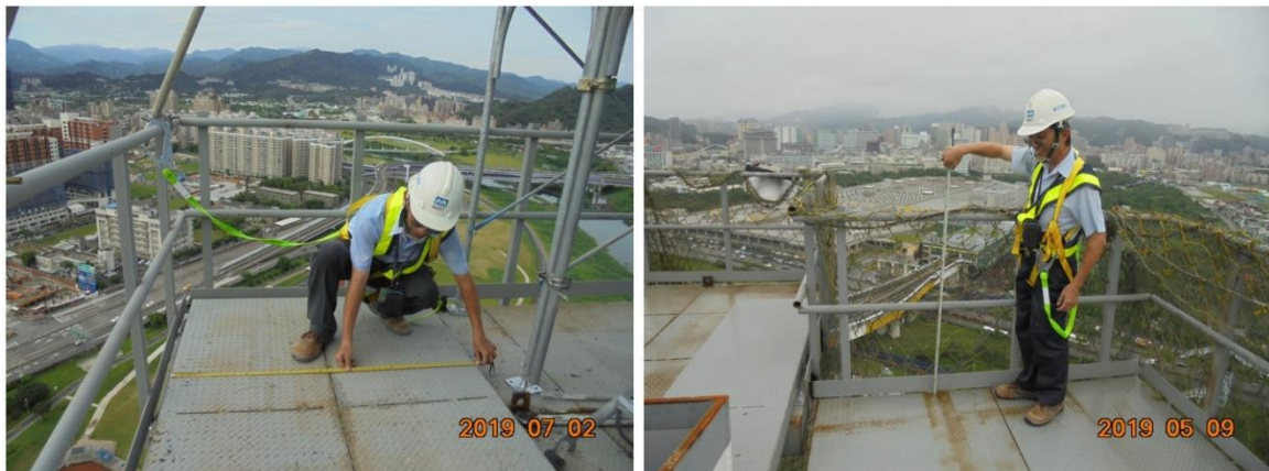
173 174 Figure 7: The inspection of the temporary working platform by the corresponding author
