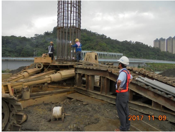
257 Figure 15: The construction of the 2m-diameter piles supervised by the corresponding author.
